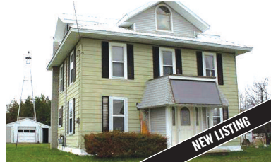
1075 N LIMITS STREET, MANCERLONA Here's your chance to own a home built in the early 1900's with 7 BR and 2 1/2 BA located just outside the city limits.
